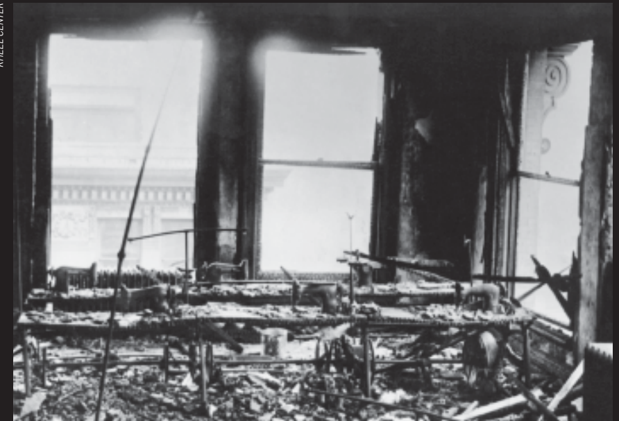
The scope and tragedy of the Triangle Shirtwaist Factory fire was apparent from its aftermath, as shown in this photo of the 10th floor work area.
