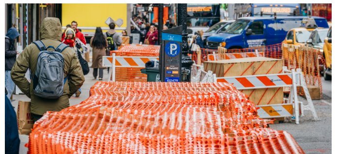
Photos of infrastructural conditions along Eighth Avenue
