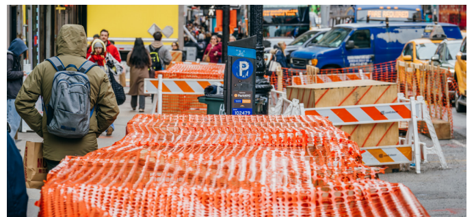
Photos of infrastructural conditions along Eighth Avenue
